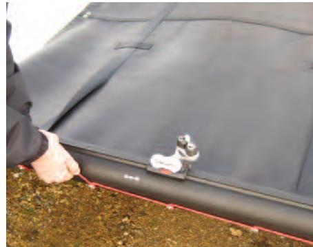
G. With the tail of the rope, feed under beam, (10) loop it over the far end of the 10mm glass fibre rod and then (11) back under the beam.
